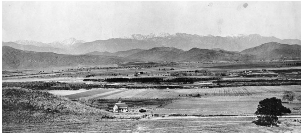
Figure 6. Glendale and environs ca.1870s. Source: Los Angeles Public Library Photo Collection.
