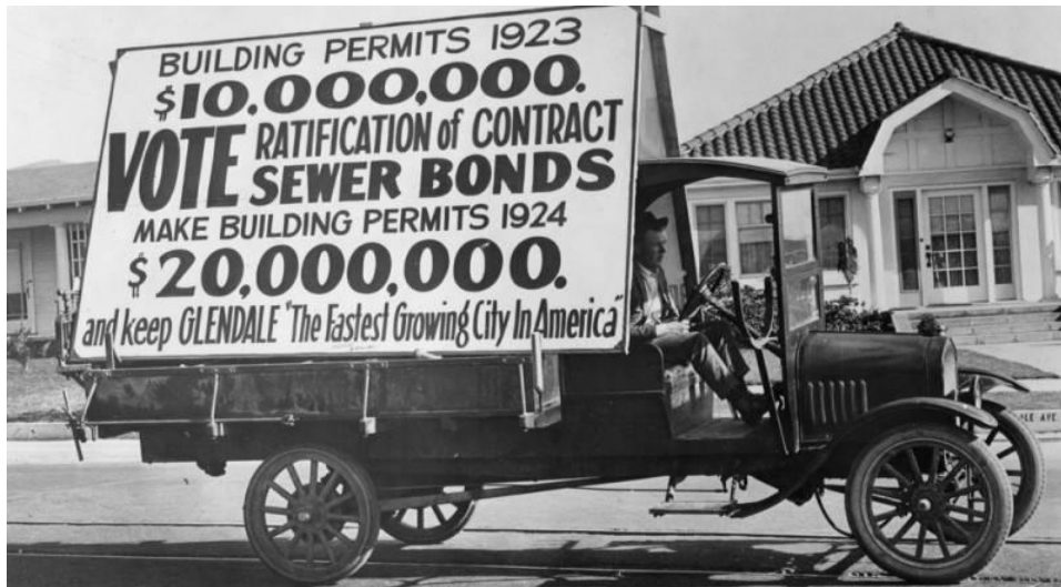
Figure 15. Truck sign touting Glendale’s growth, ca. 1923. Source: Los Angeles Public Library Photo Collection.
