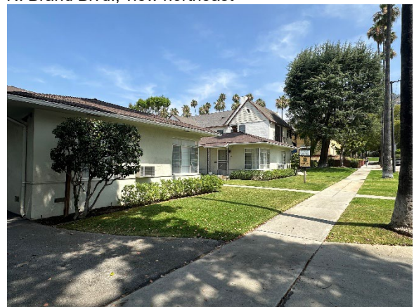
N. Brand Blvd., view northwest
