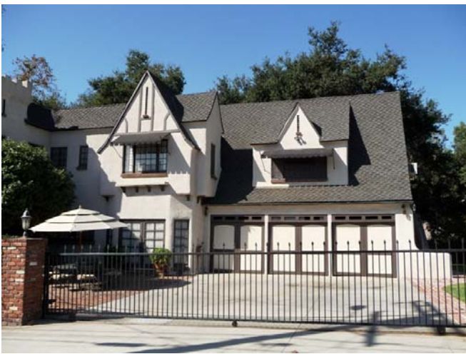
Image 4. Side (east) elevation and garage, view west. ARG, October 2014.
