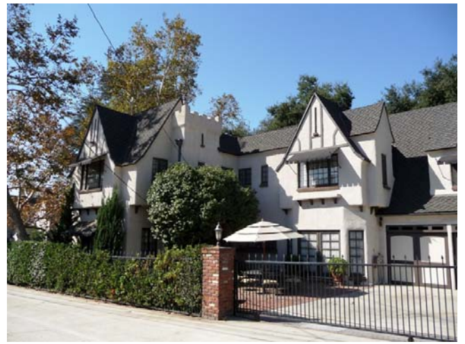
Image 3. Side (east) elevation, view southwest. ARG, October 2014.
