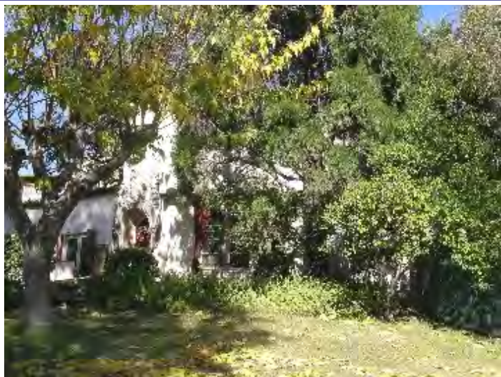
Description: South facade, north view Photo Date: 12/27/2007
