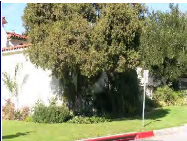
Description: South facade, north view. Photo Date: 12/27/2007
