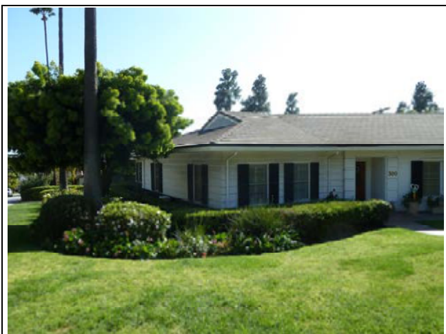
Front and side elevation, view to south, 3/27/2012
