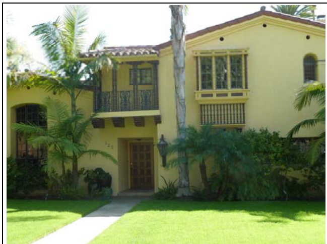
Front elevation, view to north, 3/27/2012
