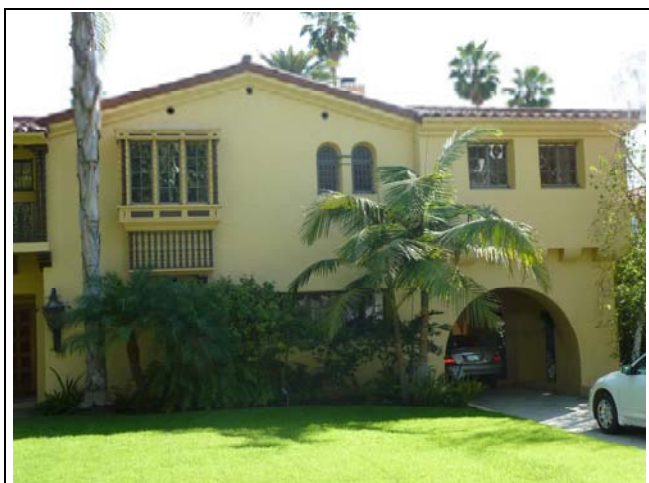
Front elevation, view to north, 3/27/2012
