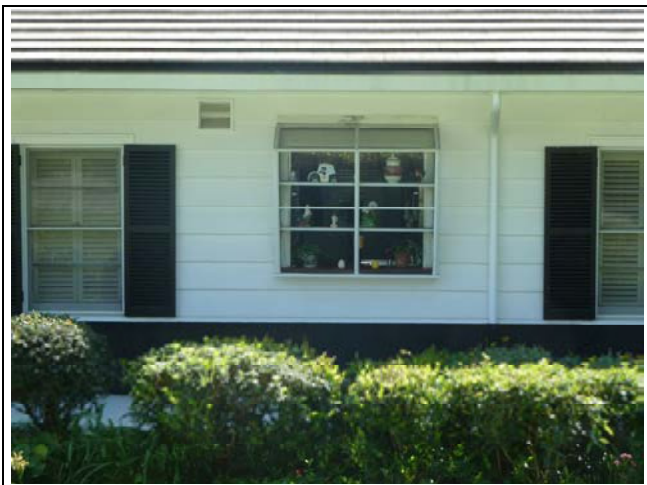
Detail of greenhouse window, view to south, 3/27/2012
